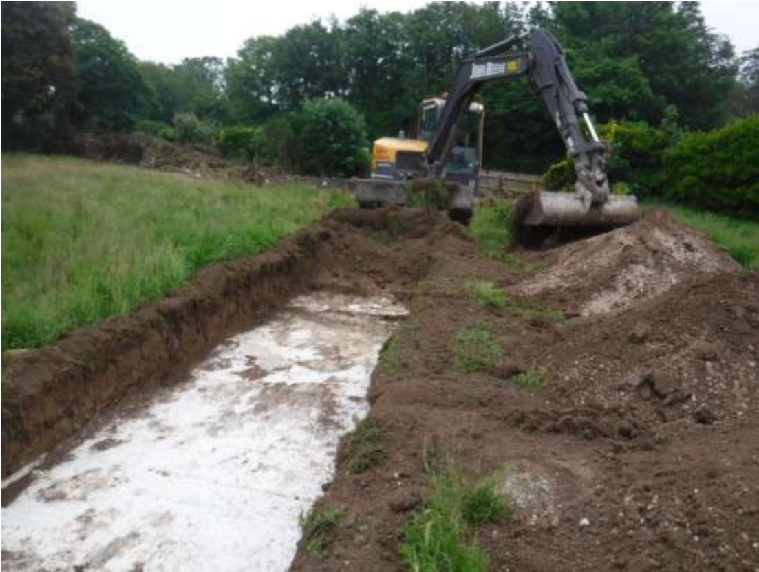
Plate 1 Opening of the Trenches
