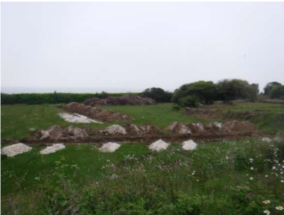
Plate 2 General view of trenches and terracing of the site
